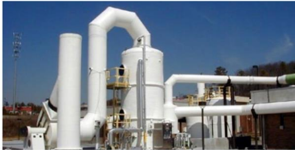
Scrubbing apparatus utilized in recovery of useful substances from gases.
